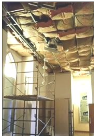
Repairs are underway in the foyer and sanctuary after water damage occurred on Jan. 2
